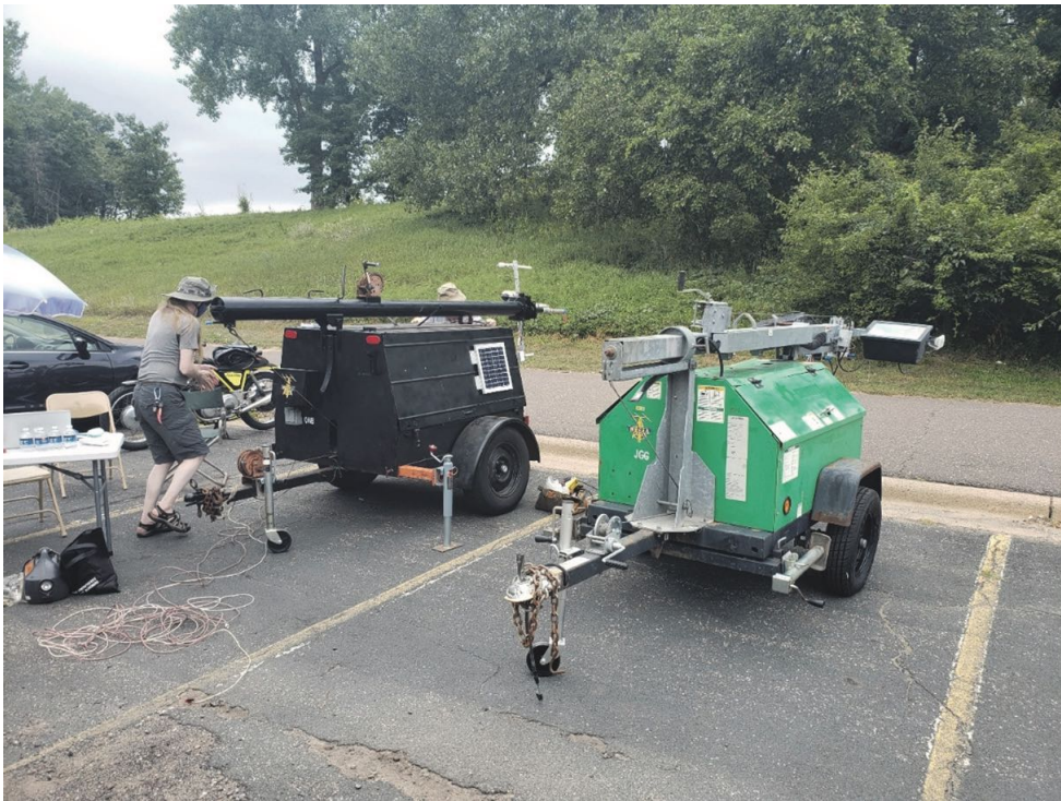
Trailer #1 (L) and #8 (R) “Jolly Green Generator” being setup at Hams in the Park here for mesh interop testing.
